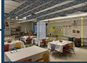
8'-10" to underside of steel structure (very limited space above existing ceiling level)
