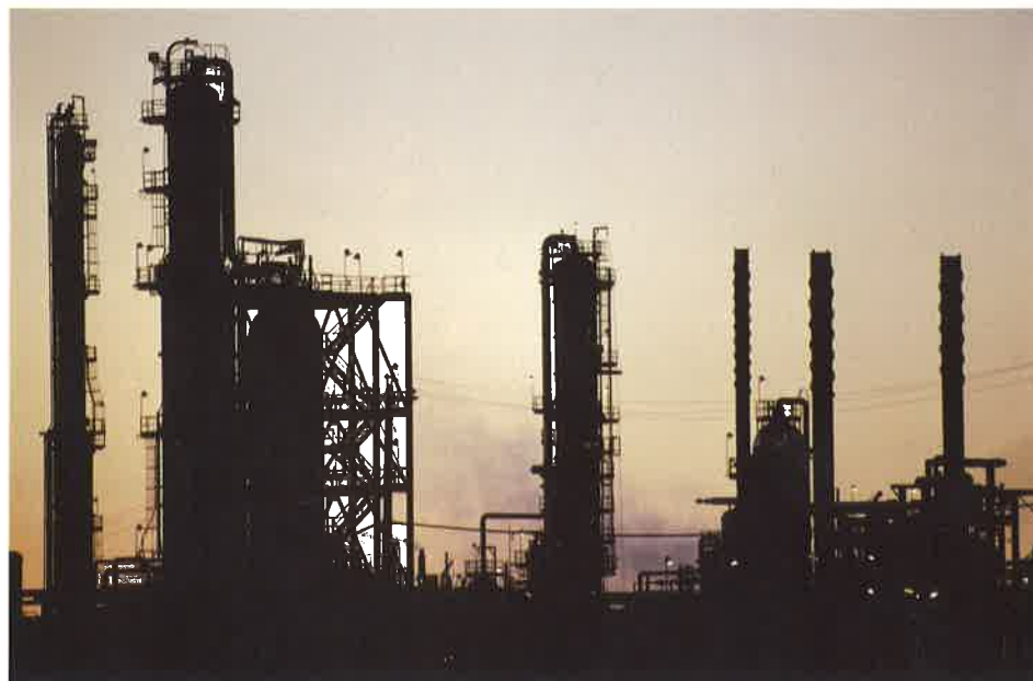
The air pollution from this oil refinery can eventually lead to water pollution.
