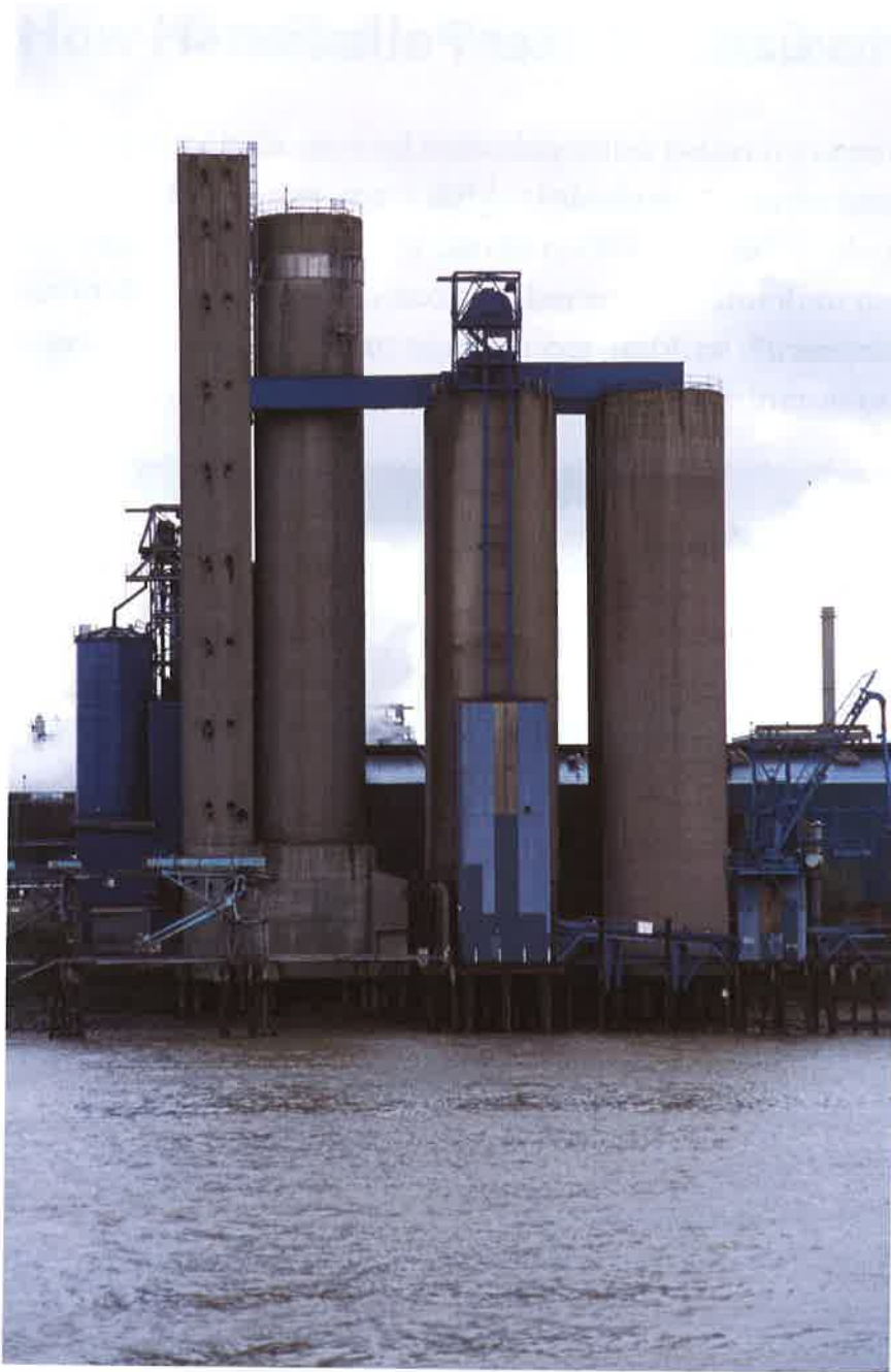
Many factories are located near bodies of surface water.
